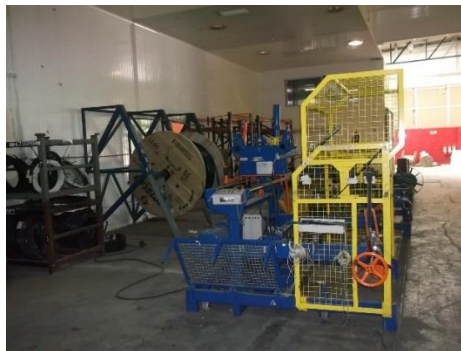
Figure 5 Cutting cables area
